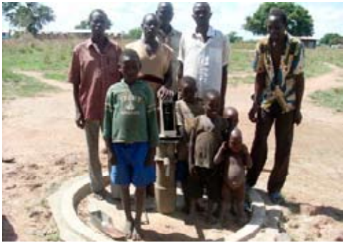
Adwir borehole before repair with the community.
