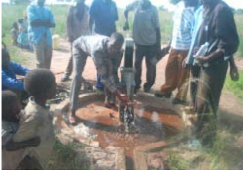
Project coordinator testing water after repair as the community looks on.
