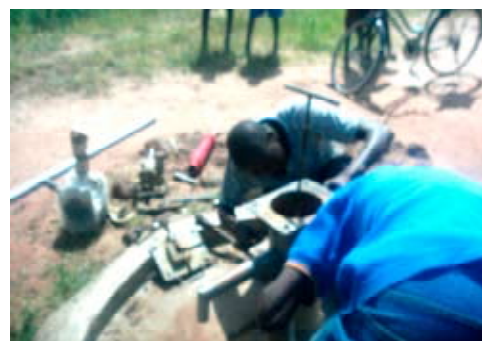
Adwir borehole during repair; Mr. Fred Okjuka, Engineer, and his Staff.
