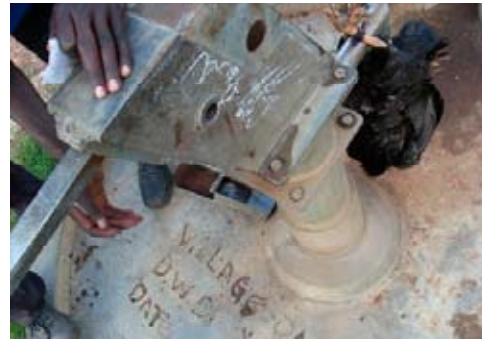
Omoro borehole before repair.
